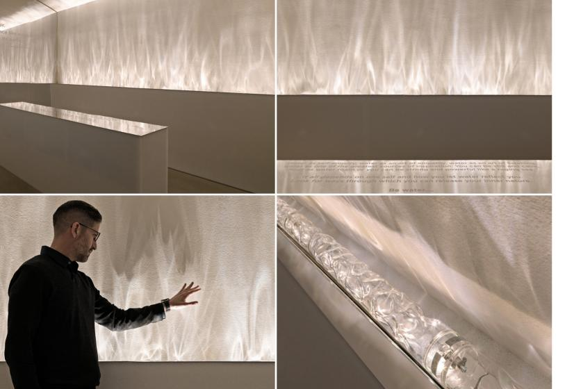
We came up with a recessed lamp within a light cove. It is a linear modular LED lamp. One single motor can rotate a glass cylinder, or two, or three...up to five, with traction, achieving any wall length.
